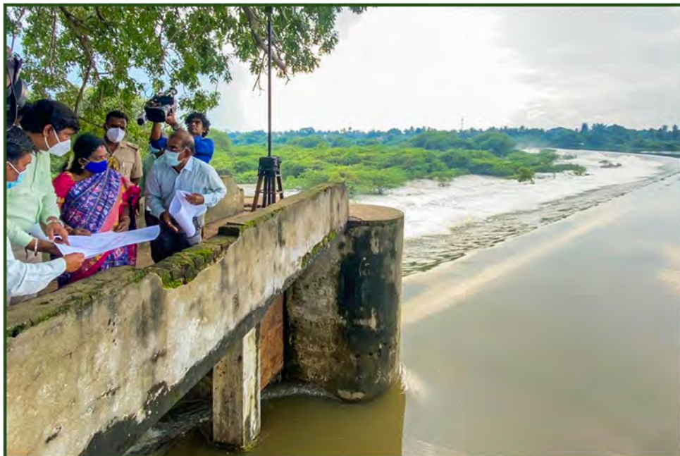
Inspection at Pilliyarkuppam Basin Dam
