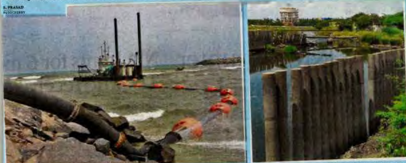
Protecting environment: Floating pipelines laid near the sea mouth at Thengalithittu fishing harbour; (right) the confluence point of the Grand canal and Uppar Canal at Vambakeerapalayam. T. SINGARAVELU
